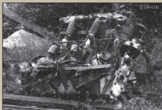
A Benz Bz.IIIa engine lies abandoned following the Armistice. Note the joined carb intake pipes (E4).
